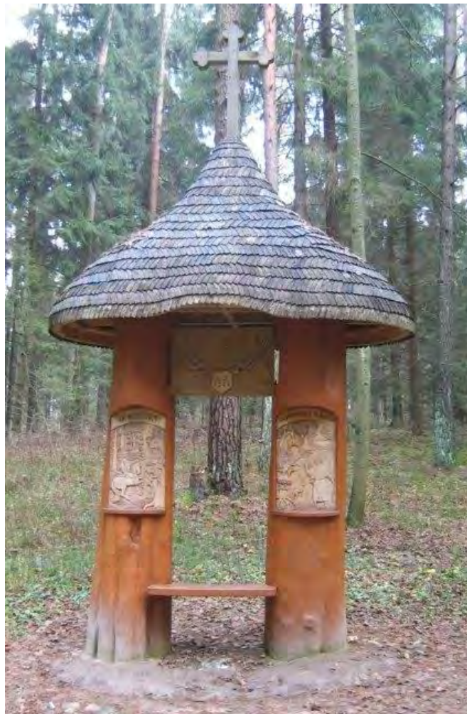
Silvarium, Poczopek, Krynki Forest Inspectorate, Podlasie, the chapel of St. Hubert and St. Eustace Placidus, Source: private picture
