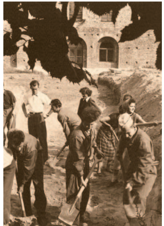
Students of the Medical Academy doing cleaning works in front of a new Dormitory
